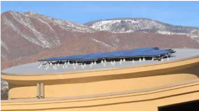
Solar panels installed on the planetarium roof in January 2016. The white mounts not attached to solar panels show where additional panels are needed. Photo by Bob Walker.
