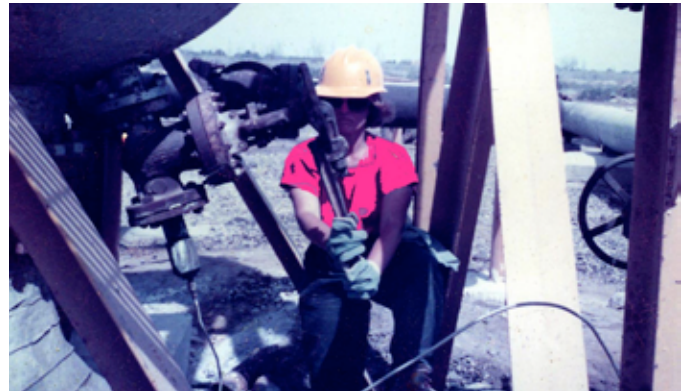
Cathy Goff swings a big wrench on production well at Cerro Prieto geothermal field, Mexico.
